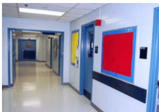
New paint and floor tiles give the autopsy suite a fresh new look.
